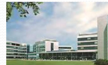
SAP Headquarters Walldorf (Germany) - 2007
